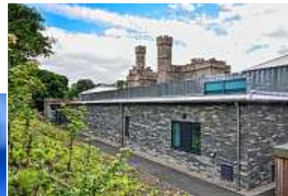
By using the principles of thermal mass and through the choice of traditional materials, the design of the new extension helps to control the temperature and humidity naturally. Pictures: John MacLean Photography
