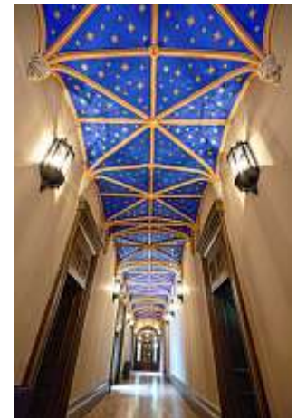
Using drawings by the original architect who first designed the castle in the 1840s for Sir James Matheson, conservation architects were able to reinstate features such as the plaster vaulting and gold stars on a blue background on the hall ceiling.
