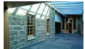
Linking the castle with the new museum, the glazed covered courtyard blends the old with the new.
