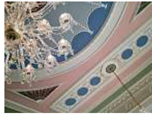
After: using traditional paint techniques, the remarkable Victorian and early 20th decorative schemes have been restored in the ballroom.
